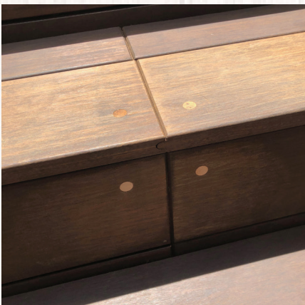
Finish as per Diagram "A" using wood Plugs
